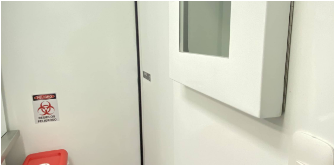
Biosafe zone detail: the combination of biological hazard signage, hazardous waste container, and sample transfer window defines the rigor of a Class 2 molecular diagnostic laboratory.
